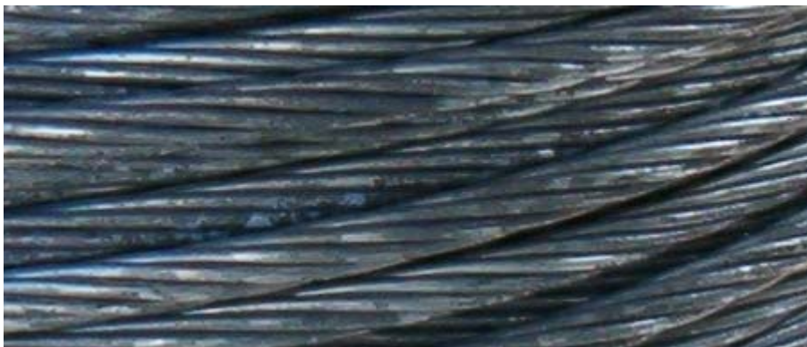
Figure 3. Oxidation on a conductor.
